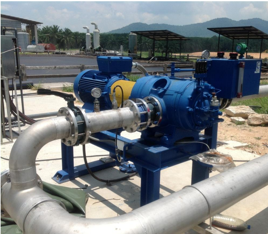
First "Mapro" Rotary vane Gas Compressor In Thailand for Palm Oil Bio-gas Plant
